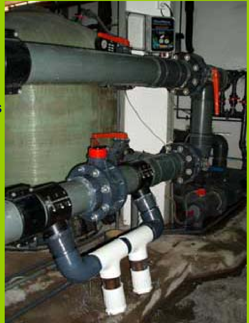
Ionization (desinfection) with 2 copper/silver electrodes.
