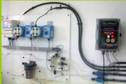
Right: control box for electrodes. Left: control of pH and redox
