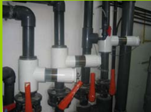
3 copper/silver electrodes
